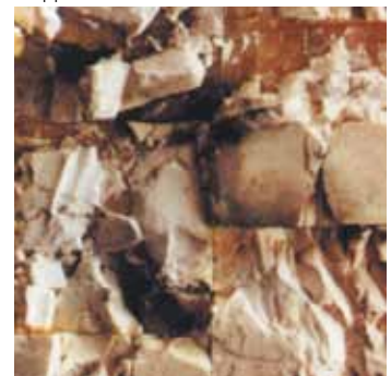
Cracked ceramic caused by fragment fire
